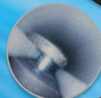
Low cost borescope through-the-scope image
